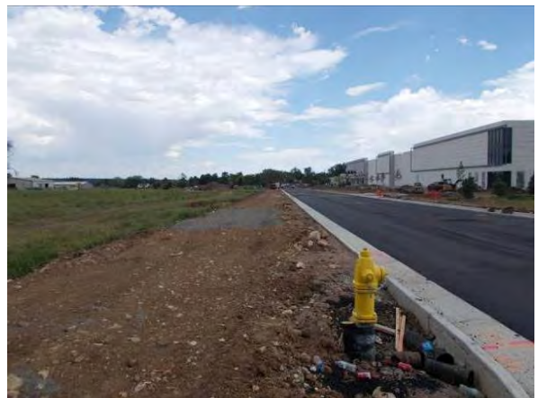
Photo #6 View along southern site boundary (eastern portion of the site). View to the east.
