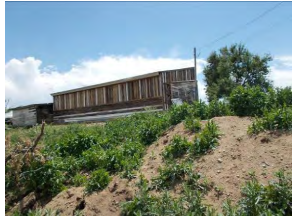
Photo #20 Overview of out-buildings observed at 6710 Indiana Street property (Parcel 39-062-00-009). View to the south.
