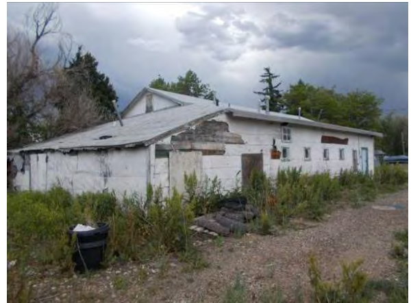
Photo #28 View of out-building on the northwestern portion of the 6730 Indiana Street property (Parcel 39-062-00-001). View to the southeast.
