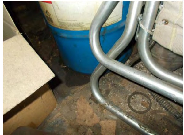
Photo #68 View of staining at the base of the 120-lb. keg of grease observed in the office/parts room (Observed on June 18, 2020).
