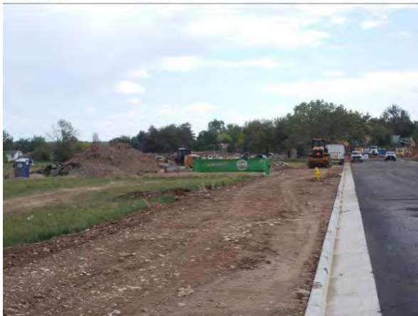
Photo #35 Overview of vacant site property (with construction staging area) 14355 West 67 th Avenue (Parcel 39-063-02-002). View to the south.
