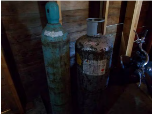
Photo #93 View of compressed gas cylinders observed in garage/storage building (Observed June 30, 2020).
