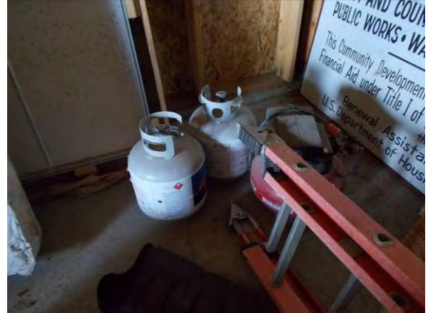
Photo #92 View of the propane canisters observed in garage/storage building (Observed June 30, 2020).
