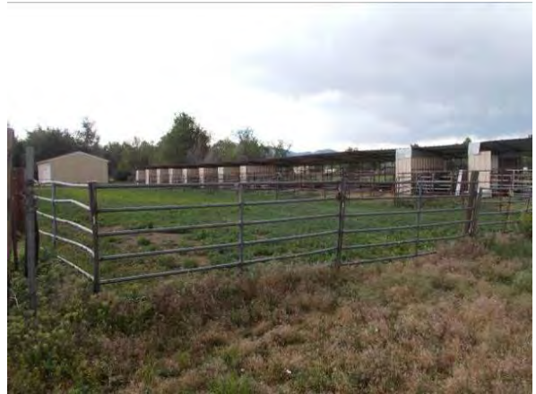
Photo #14 Overview of vacant stables observed on northern portion 6702 Indiana Street property (Parcel 39-063-00-003). View to the northwest.
