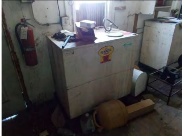
Photo #63 View of two hydraulic oil ASTs observed along the western wall of the office/parts room. (Observed on June 18, 2020).
