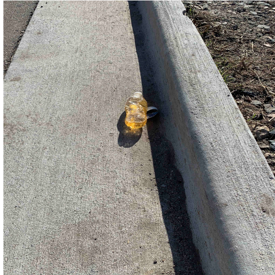
Urine bottle 2 was full and in storm drainage gutter
