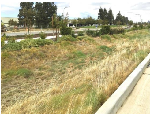
Native Grass Bioswale
