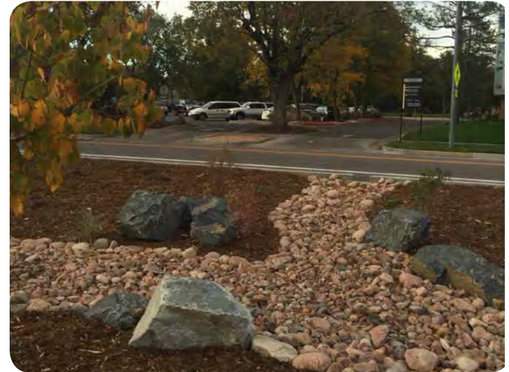
Storm Water Best Management Practices: Rain gardens that slow down and filter storm water with landscape.
