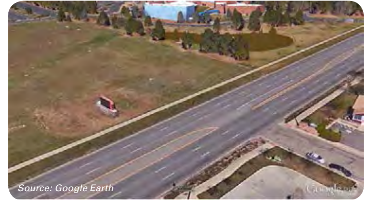
Existing conditions along Wadsworth Boulevard at the Arvada Center for the Arts.
